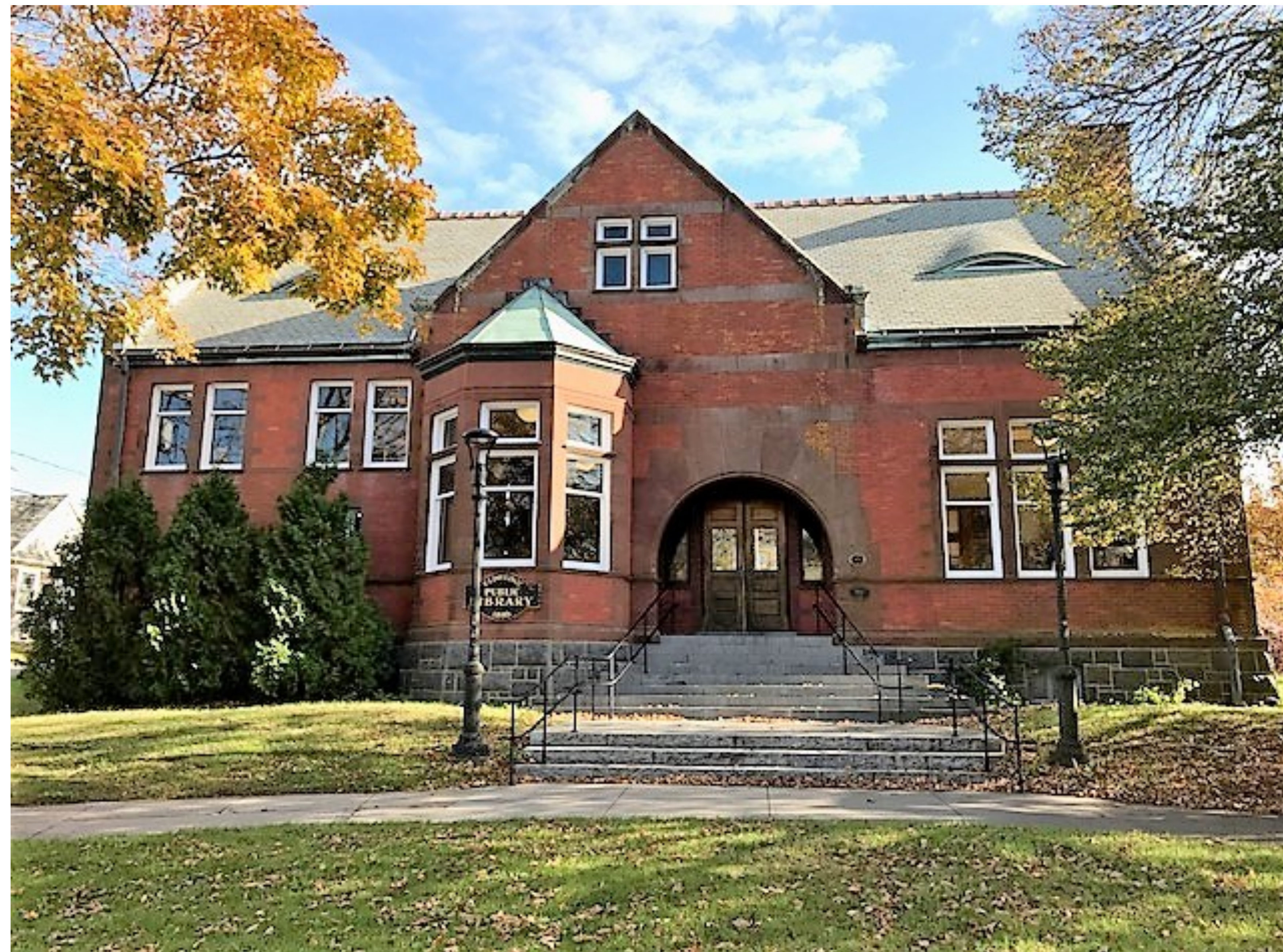
564 Main Street - Eldredge Public Library Owner: Town of Chatham
